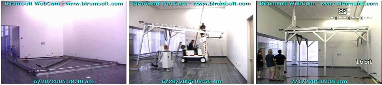
Figure 2: Image stills from time-lapse recording of the rig's construction
